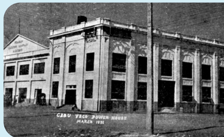
POWERING A GROWING CITY. When it began operations in the early 1900s, the Visayan Electric Company or VECO ran and maintained its own diesel energy generation plant (above photo) and electricity distribution network serving residential and commercial consumers in Cebu City.
